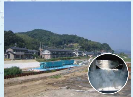
Polluted Water Treatment and Heavy Metal Removal
