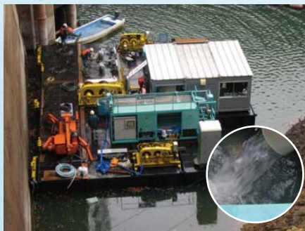
Polluted Water Treatment in Wire-saw Operation
